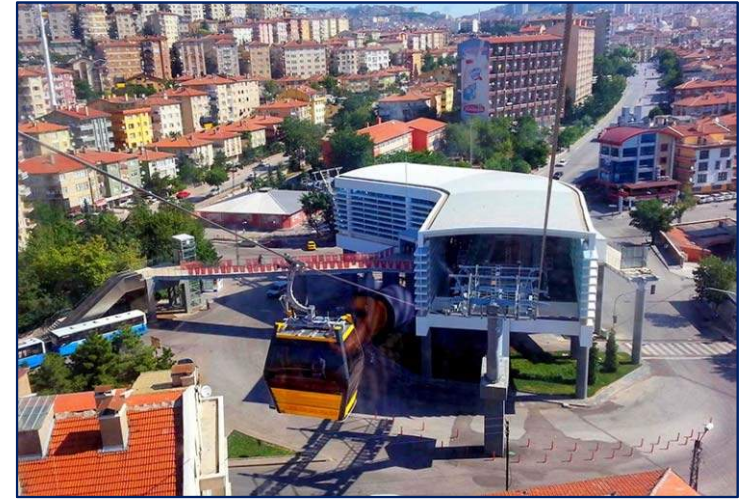
Ankara, Yenimahalle-Şentepe cable car line
